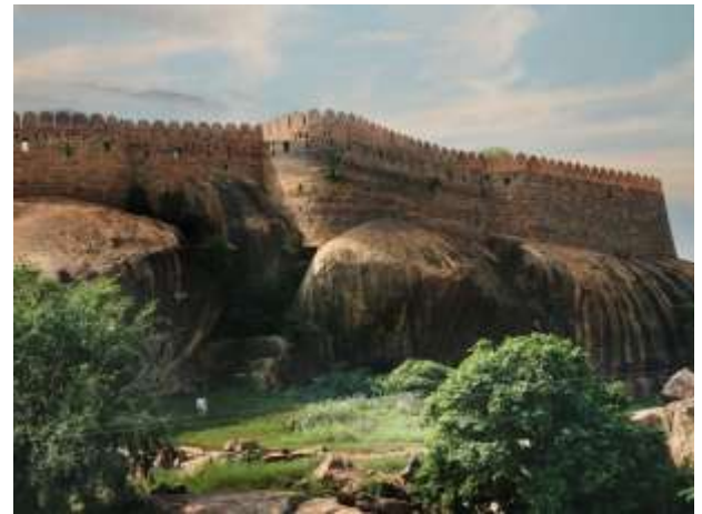
Fig. 3. Fortification walls of Tirumayam Fort rising directly from the natural granite scarp, illustrating the integration of constructed masonry with bedrock terrain.
