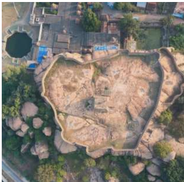
Fig. 4. Aerial view of the fort's hilltop interior, showing the octagonal pushkarani (temple tank) at upper left alongside the fortification walls under conservation.
