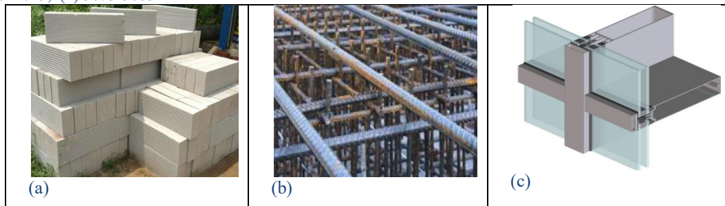
Figure 2: Material Used- (a) AAC blocks (b) Reinforcing steel, (c) Curtain wall systems
